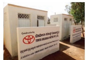
Construction of School Sanitation Units in Government Schools
